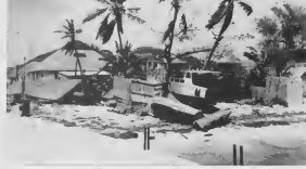
HURRICANE DAMAGE at St. Martin is shown in this dramatic photo cast in by David Vlaun. Cracking. Palm trees are disheated, a boat thrown up on dry land, and various buildings smashed.
